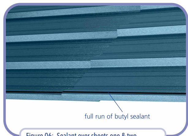
Figure 06: Sealant over sheets one & two
